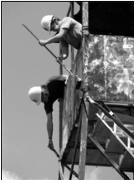
August and September of 2002: Work on the fire tower continues, including: damaged roof panel removed and replaced with reconditioned panel; fencing replaced and secured with staples/wire; water bars installed above cedar step work to reroute water; 3 tons of stone (one ton flown and two tons hauled by hikers) on summit being used for soil erosion prevention; summit areas seeded and brushed in; and a new cedar ceiling installed in tower cab.
